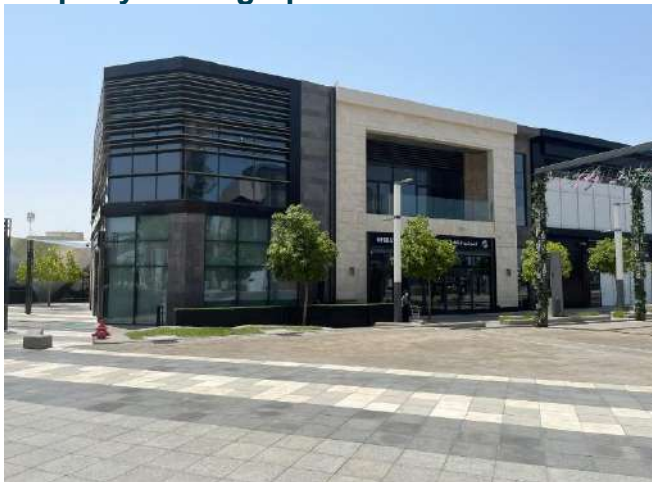
Source: JLL Inspection 2024
