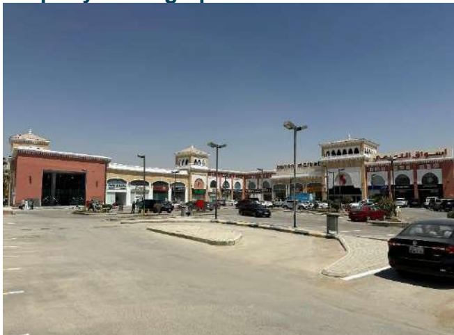
Source: JLL Inspection 2024
