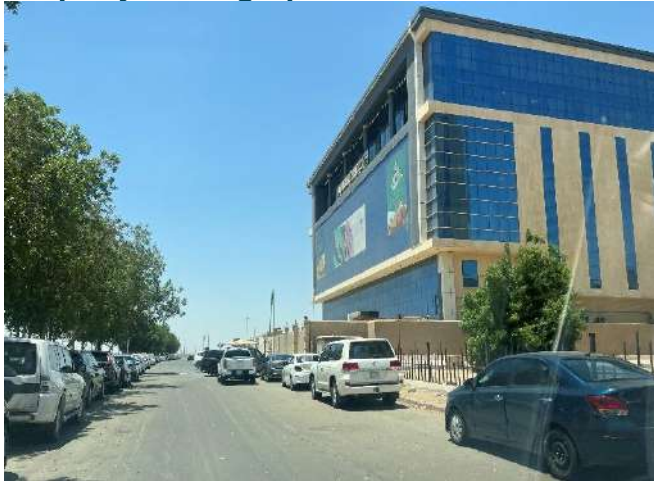
Source: JLL Inspection 2024
