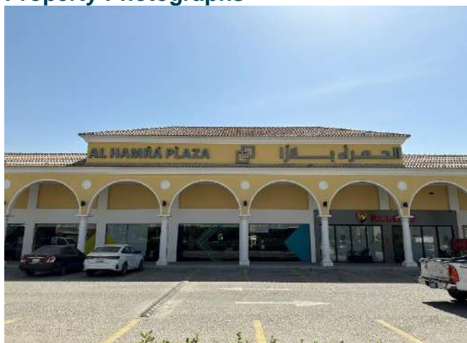
Source: JLL Inspection 2024
