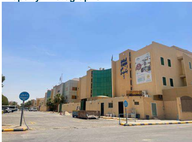
Source: JLL Inspection 2024
