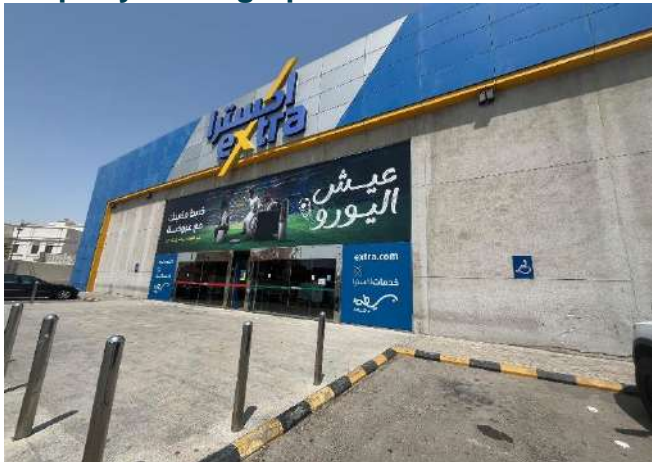
Source: JLL Inspection 2024
