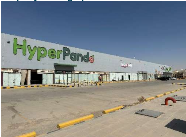
Source: JLL Inspection 2024
