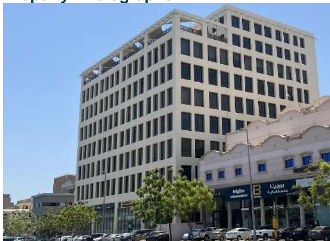
Source: JLL Inspection 2024
