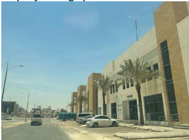
Source: JLL Inspection 2024
