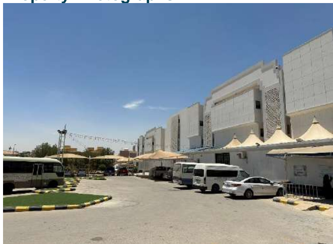
Source: JLL Inspection 2024
