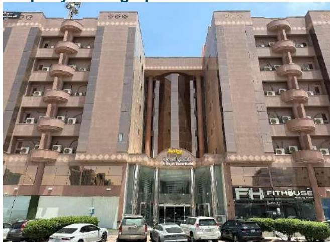
Source: JLL Inspection 2024
