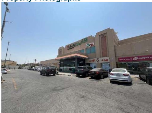
Source: JLL Inspection 2024
