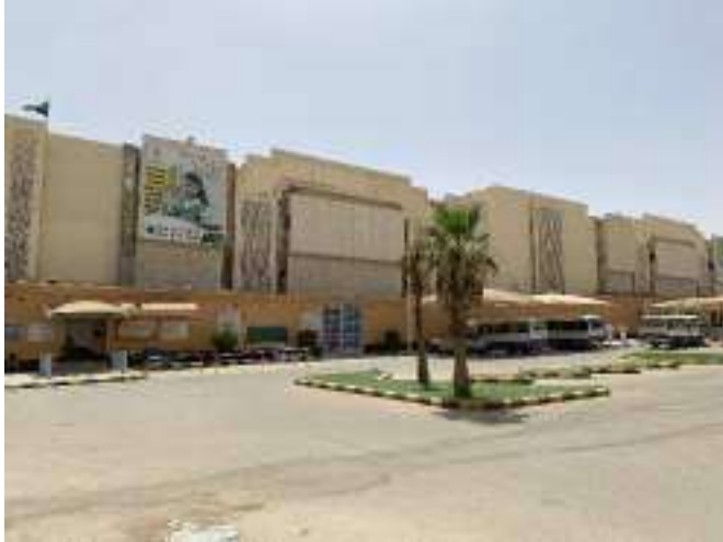
Source: JLL Inspection 2023
