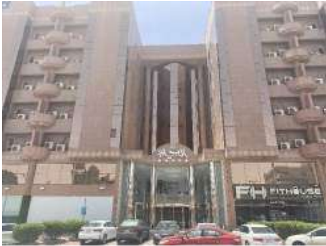
Source: JLL Inspection 2023
