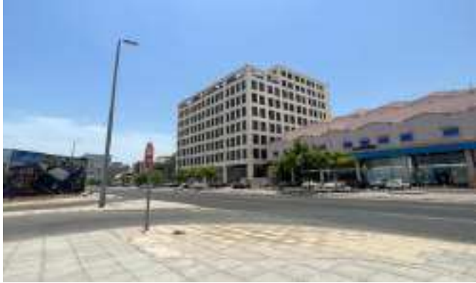
Source: JLL Inspection 2023
