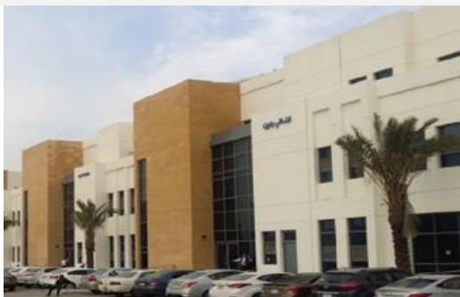
Dar Al Baraa School
