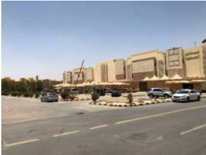
Source: JLL Inspection 2022
