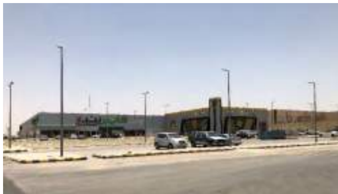
Source: JLL Inspection 2022
