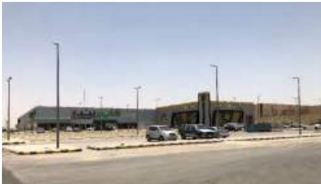
Source: JLL Inspection 2022
